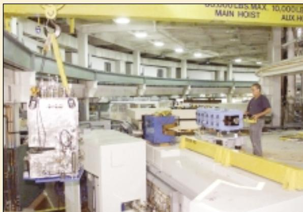
One of three superbends being lifted over the shielding wall just before installation in the storage ring, August 20, 2001.
