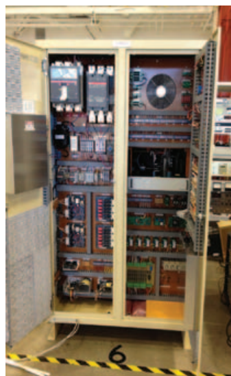
Left: New storage-ring bend-magnet supply, operational since March 2013. Right: One of 48 new sextupole magnets installed in the storage ring as part of the brightness upgrade.
