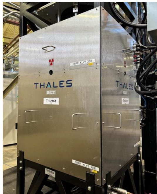
Fig. 13. The operational Thales klystron pictured above is an essential part of the ALS storage-ring radio frequency system. Sourcing of these original equipment manufacturer units or alternatives requires special attention to the supply chain.
